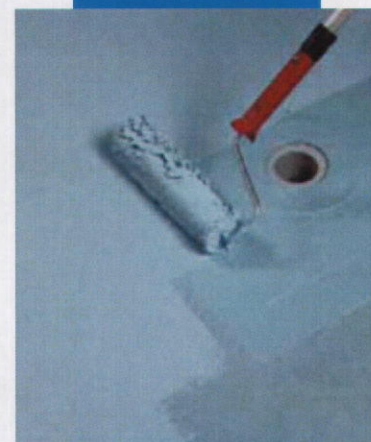
Application by roller of Mapelastic® AquaDefense second coat
