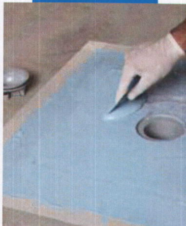
Impregnating Drain Vertical fabric with Mapelastic® AquaDefense
