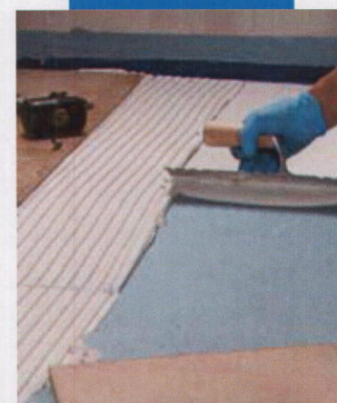
Bonding tiles on Mapelastic® AquaDefense
